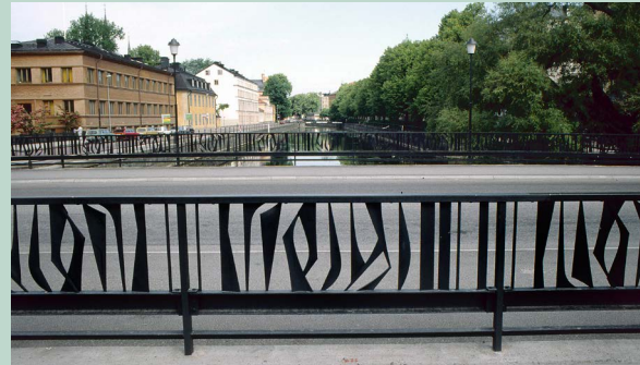
Artist: Olof Hellström Title: Variabel rapport [Variable Report] Created: 1965 Location: Islandsbron bridge Owner: Uppsala Municipality To be preserved in connection with the expansion of Uppsala Tramway
